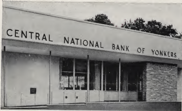
L-4: Sans-serif letters fabricated of stainless steel with black porcelain enameled recessed faces. Letters are assembled on a stainless steel channel in a free-standing manner.
